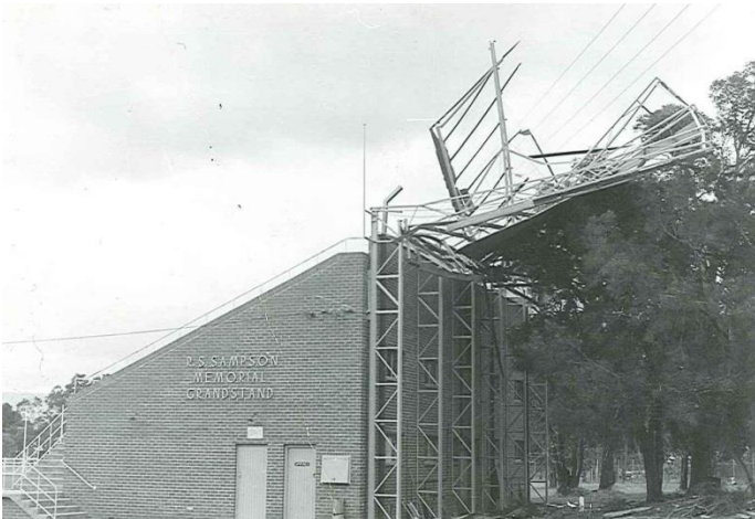
Storm damage to grandstand 1965.
