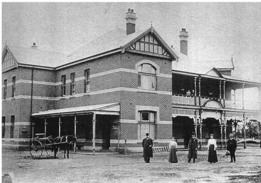
Figure 10 Gosnells Hotel, c.1910 Courtesy Heritage Inventory of Heritage Places, 1998.
