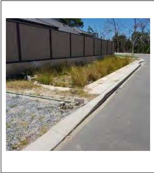
Plate 2: Example Rainwater garden in verge
