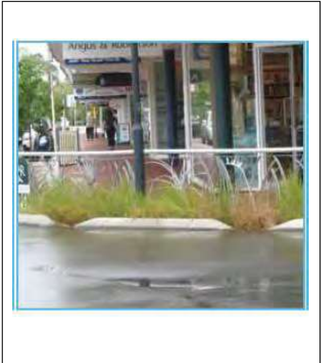
Plate 3: Roadside biofilter with split guttering
