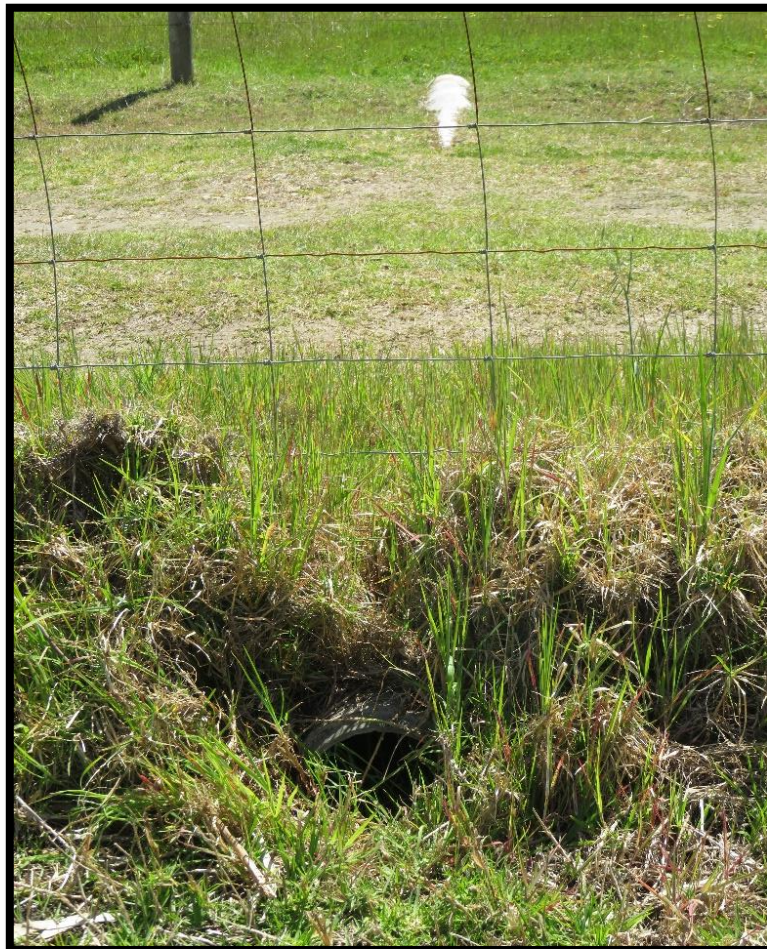
Plate 9: Pipe culvert under limestone track
