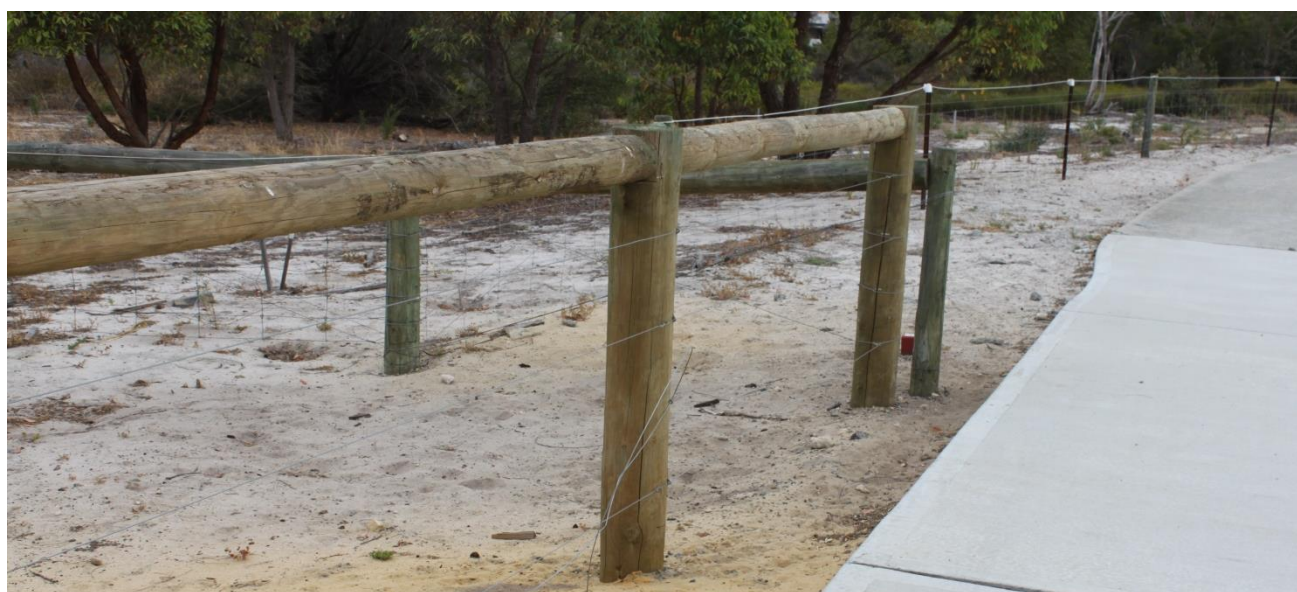
Figure 8: Post and rail fence
